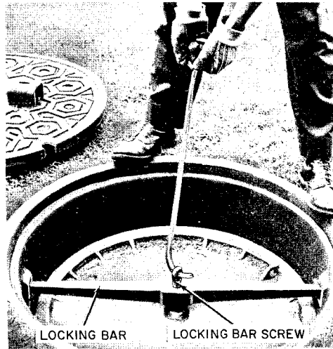
Fig. 27—♦Loosening Locking Bar Screw♦
