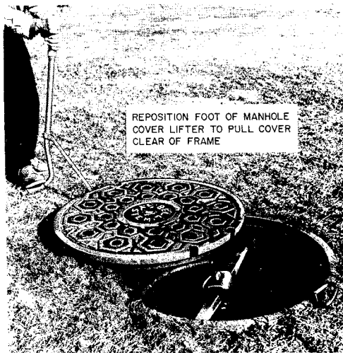
Fig. 33—Pulling Cover Clear of Frame
