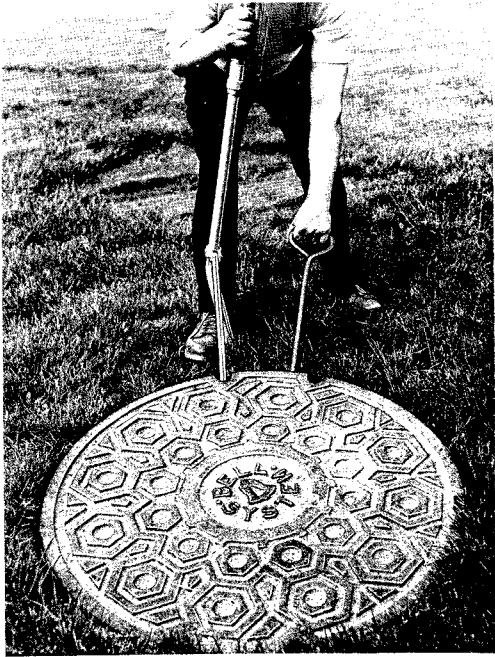
Fig. 31—Inserting B Manhole Cover Hook for Positioning on Locking Bar
