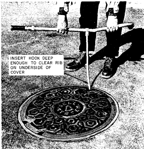
Fig. 29—Inserting PTS-49 Manhole Cover Lifter Hook Into Hook Hole
