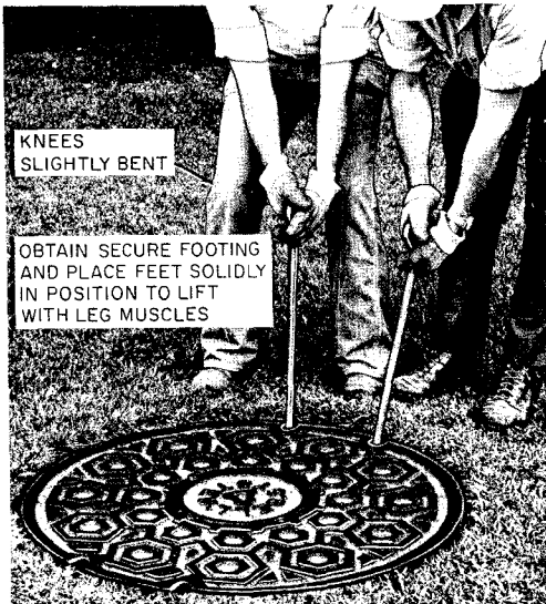
Fig. 34—Preparing to Unseat Cover—Two-Person Method
