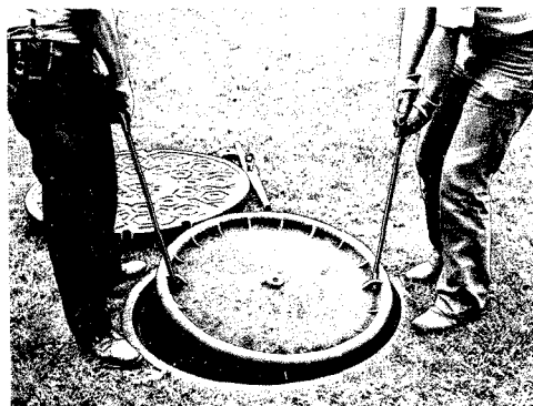
Fig. 38—Removing Inner Cover—Two-Person Method
