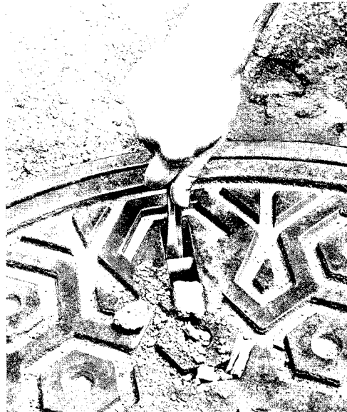
Fig. 13 - Cleaning G or H Manhole Cover Lifter Pocket
