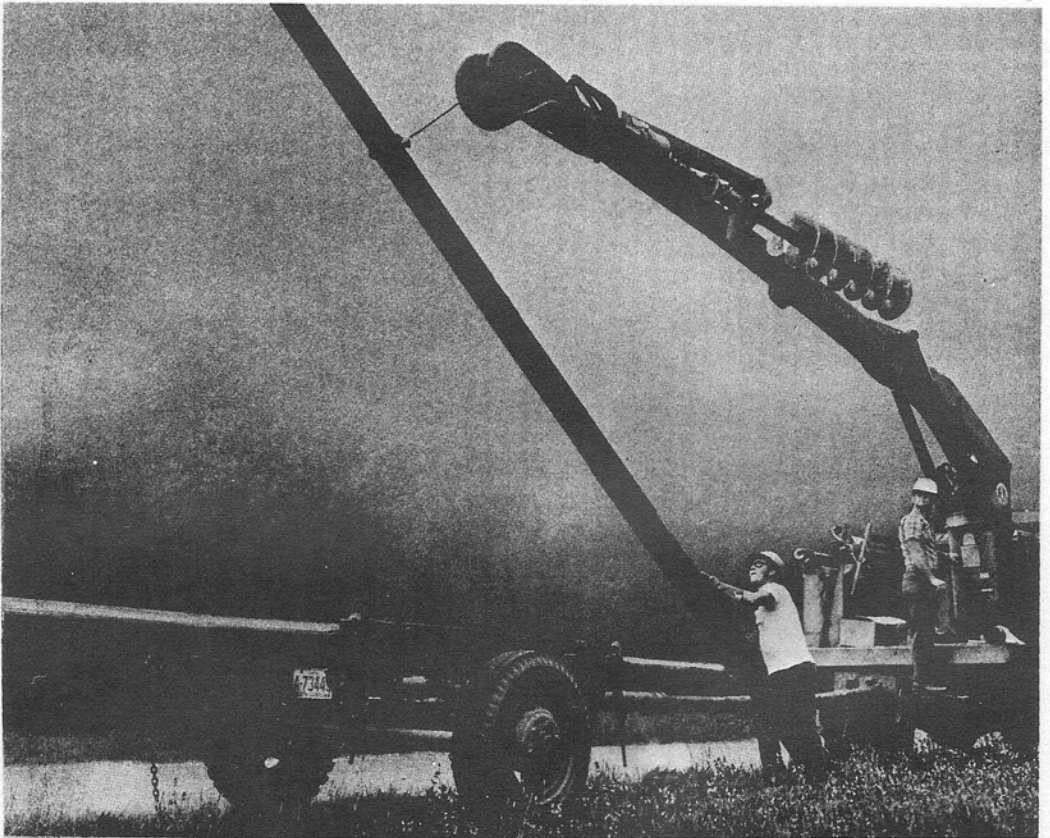
Fig. 6—Removing Single Pole in Preparation for Installation
