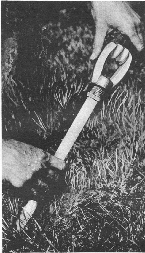
Fig. 15—Completed Anchor Installation
