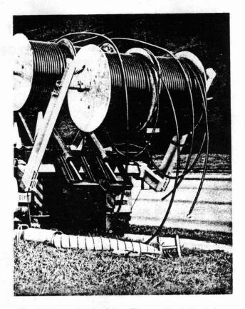
Fig. 1—Setup for Reel Handling at Feed Manhole
