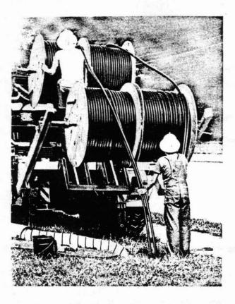
Fig. 3—Observing Innerduct as It Is Placed
