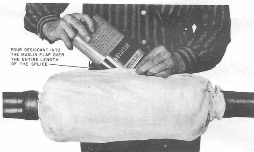
Fig. 5—Applying Desiccant to Wet Conductors
