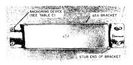
Fig. 29—45A Mounting Bracket Mounted Horizontally on Wall
