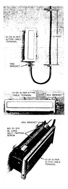
Fig. 30—Securing 10- or 16-Pair N-Type Cable Terminal to 45A Mounting Bracket
