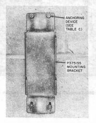
Fig. 35—P-375155 Mounting Bracket Secured To Wall
