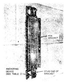
Fig. 28—45A Mounting Bracket Mounted Vertically on Wall
