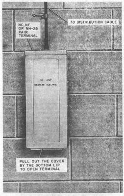
Fig. 38—Terminal Arranged for Splicing To Aerial Cable
