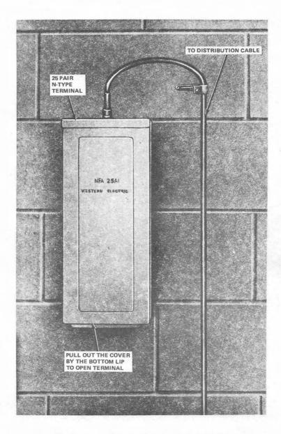
Fig. 22-Terminal Arranged for Splicing to Buried Cable
