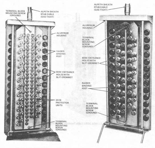
Fig. 5-NCA-25A1 Cable Terminal
