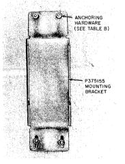
Fig. 20—P-375155 Mounting Bracket Secured to Wall
