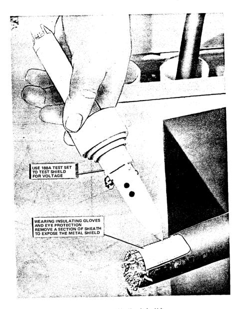
Fig. 1—Testing Cable Sheath for Voltage
