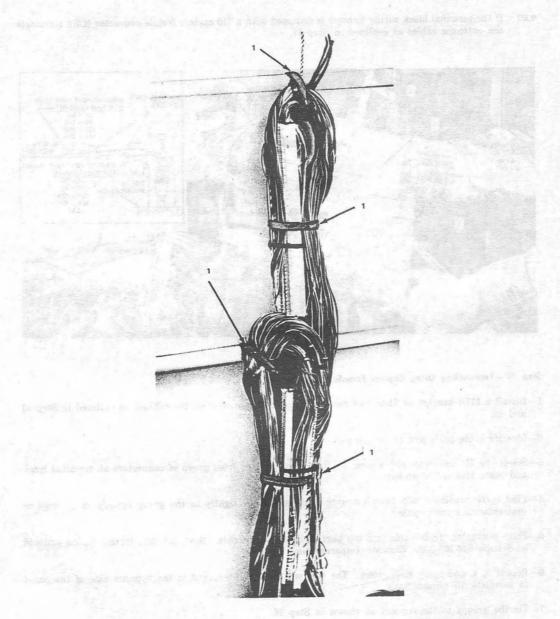
Step 16-Spliced Groups Secured to Splicing Support
