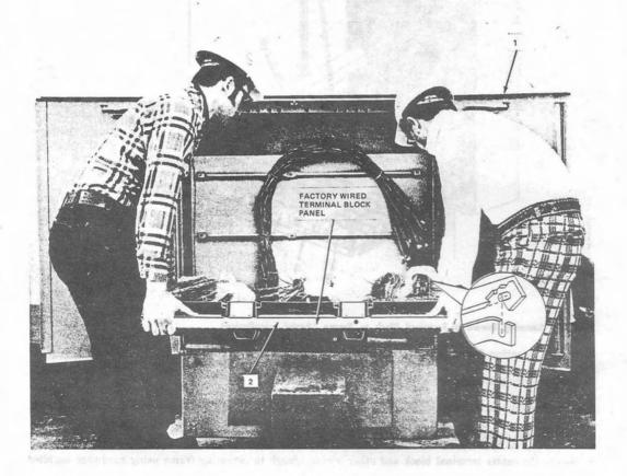
Step 13—Installation of Frame Equipped With Terminal Block
