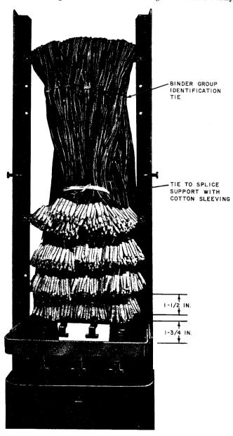
Fig. 24—Completed Splice
