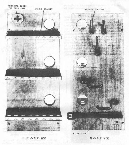
Fig. 8—M Backboard (for LE10/42 Cable Closure)
