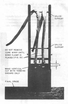
Fig. 18—Sheath Removed—Cut Ends
