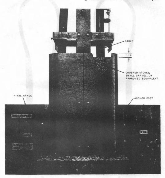
Fig. 16-LD- or LE-Type Closure Placed
