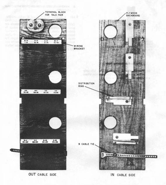
Fig. 7—L Backboard (for LE6/42 Cable Closure)
