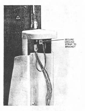
Fig. 17—Sheath Preparation for Aerial Entrance Cable
