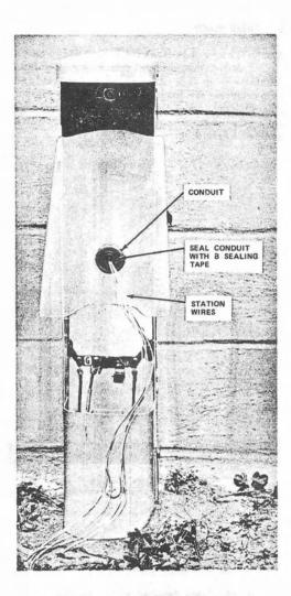
Fig. 13-PC6/48 Cable Closure-Wall Mounted
