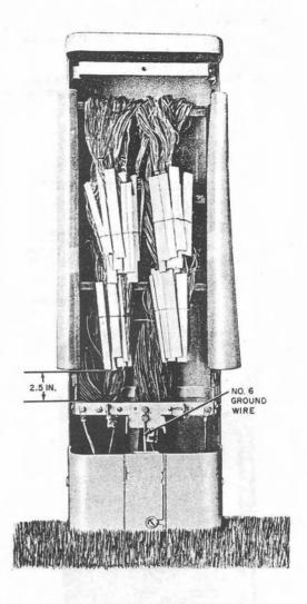
Fig. 24—Completed Splice in PC12/55 Cable Closure Using 710 Connectors
