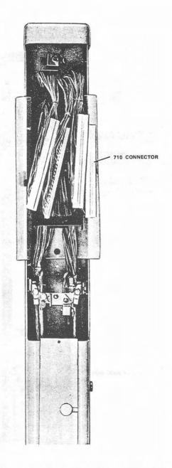
Fig. 22—Completed Splice in PC4/48 Cable Closure
