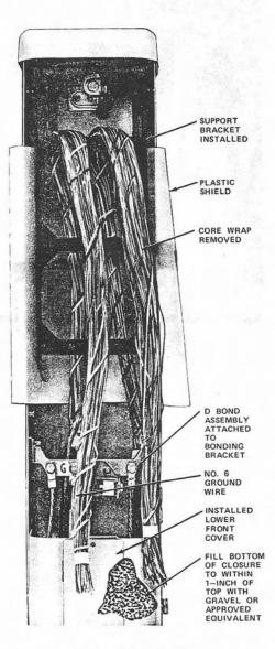
Fig. 18—Installed Cable Closure
