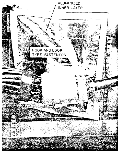
Fig. 10—KS-21822 Temporary Splice Cover
