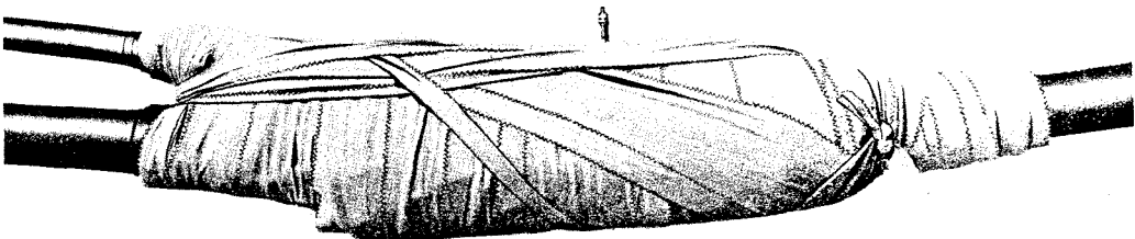
Fig. 23—Reinforcing CR Tape Cover
