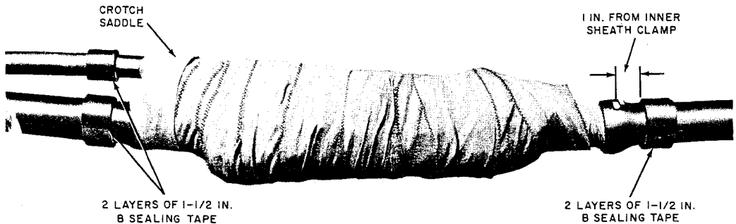
Fig. 7—Crotch Saddle and B Sealing Tape Installed (Single Use)
