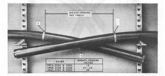
Fig. 11-Mark Cable Sheath
