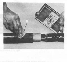
Fig. 16-Cleaning Cable Sheath
