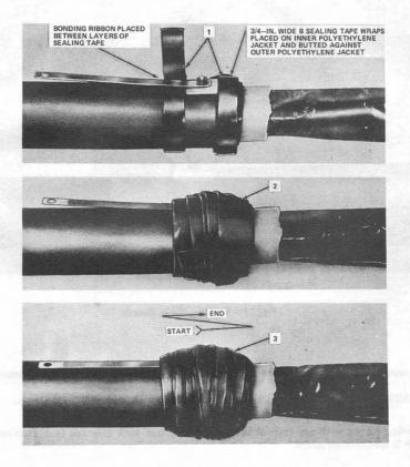
Fig. 18—Constructing Wrapped Joint
