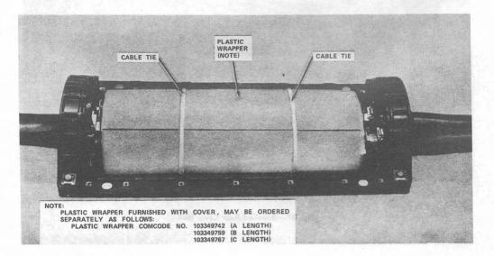
Fig. 38—Completed Splice
