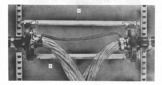
Fig. 33—Installed 819A Alignment Bar
