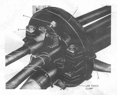
Fig. 30—installed End Plates
