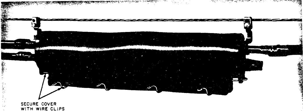
Fig. 8—Completed Installation—Normal Pull-out (Cover Placed)
