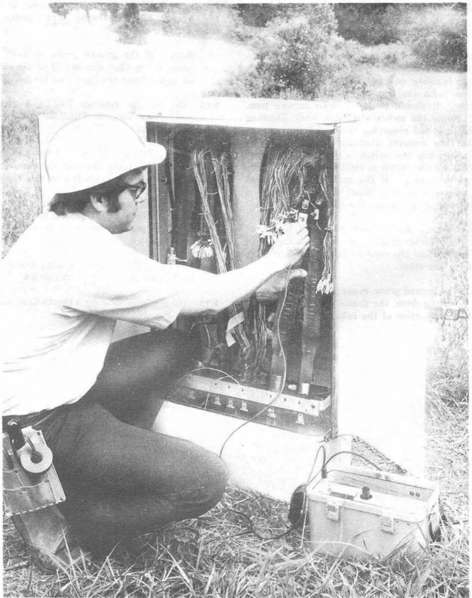
Fig. 10—Connecting Transmitter
