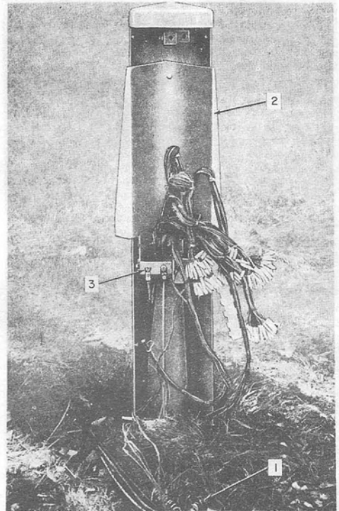
Step 94—Place Back Section of PC6/48 Cable Closure Placed In Excavation
