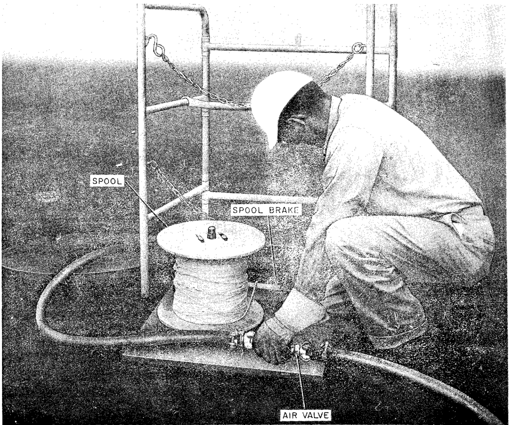
Fig. 9—Placing B Fishline from Spool
