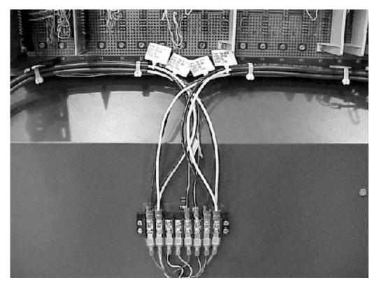
11 Connect the cables to the appropriate terminals. Refer to Figure 35 or cable tags for the connections.
