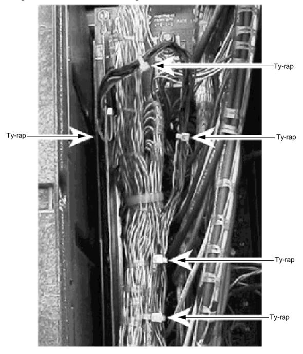
Figure 62 – NT0X26DV Cable Forming Part 1 of 3
