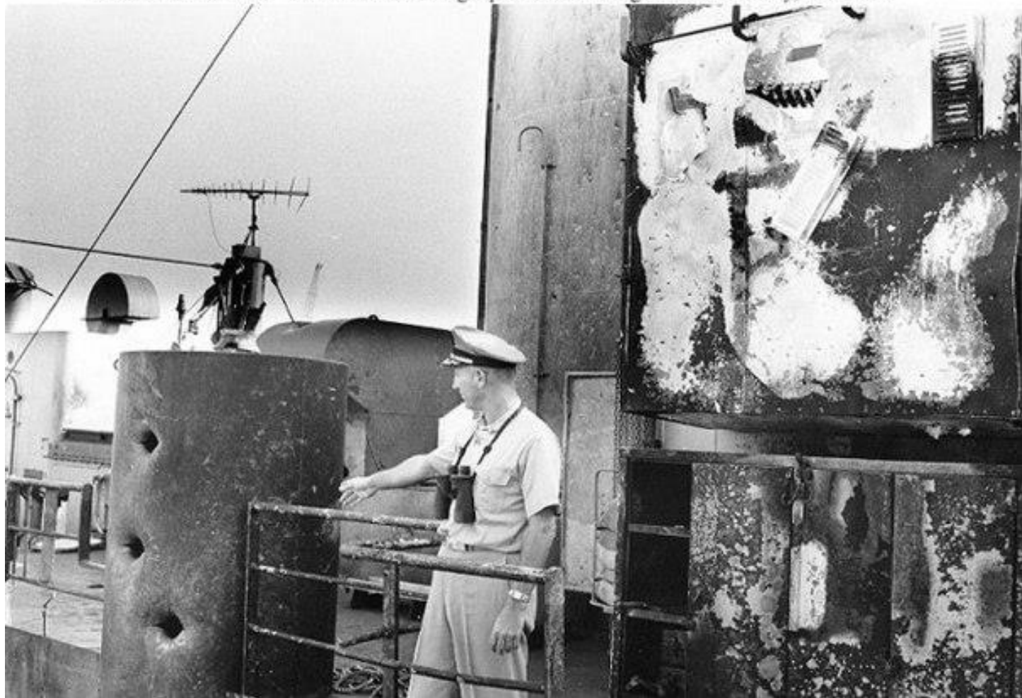
Photo # NH 97476 Cdr. W.L. McGonagle points out damage on USS Liberty, June 1967
