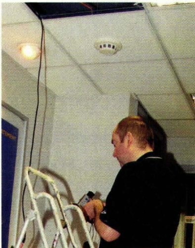
Concealing miniature video camera inside smoke detector
