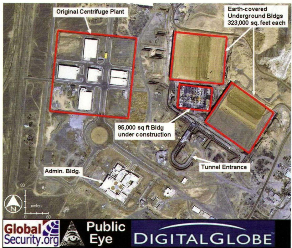
Overview of construction at Natanz as of 29 August 2002. (IMAGE SOURCE: DIGITALGLOBE)
