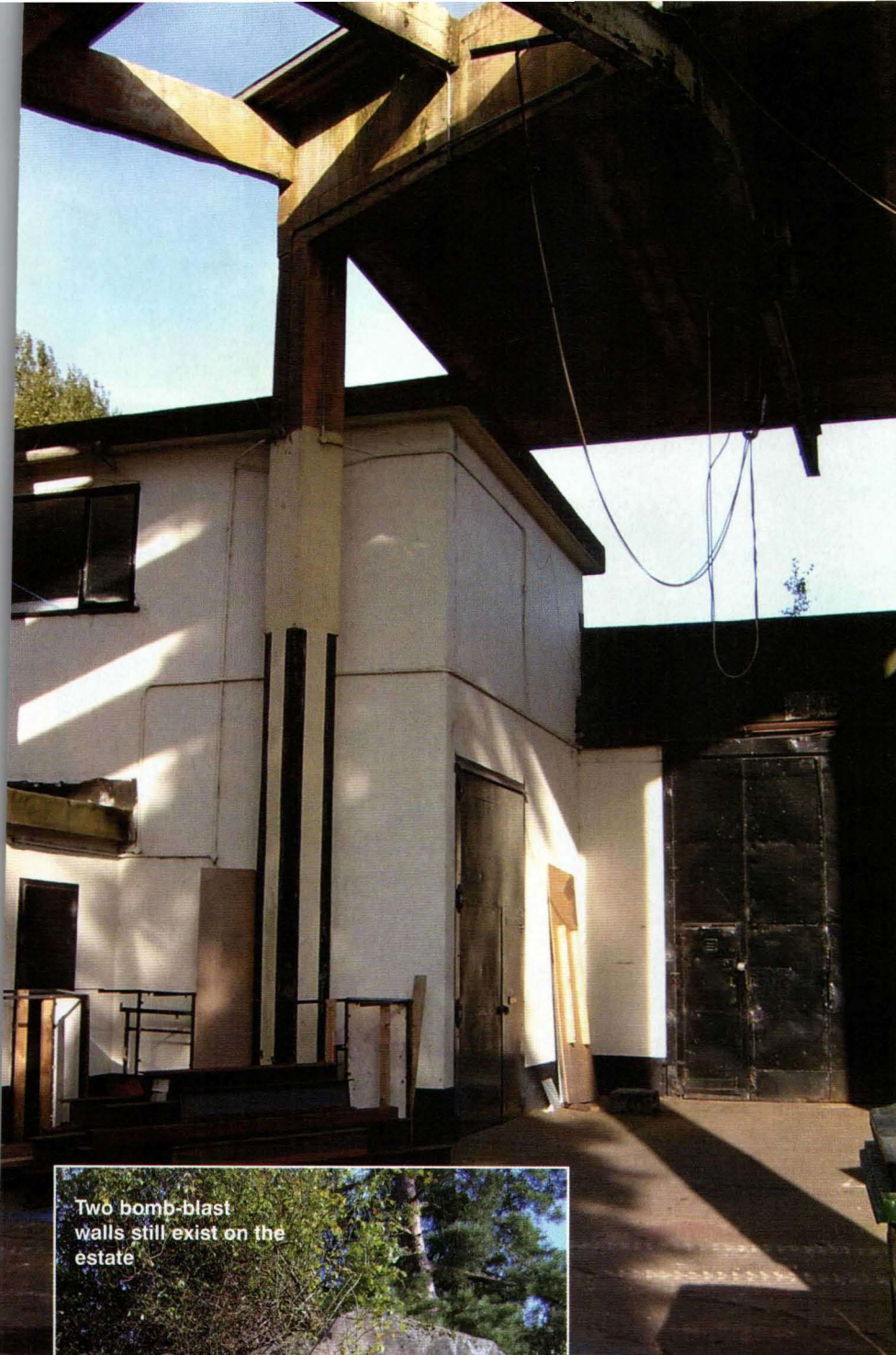
The huge hoist to remove the bomb from transporters is still evident. Behind is one of the buildings used to store the case
