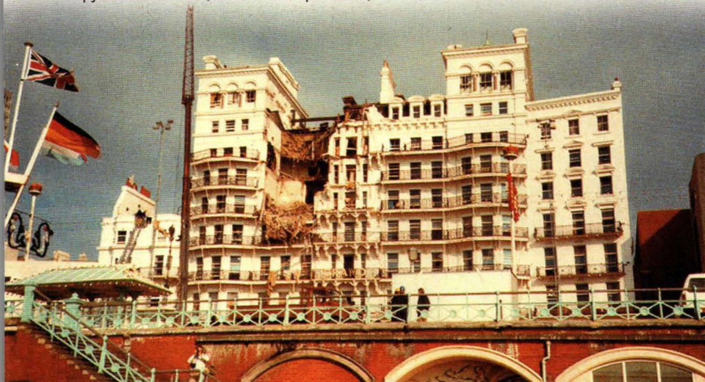
Damage to the Grand Hotel, Brighton is clearly visible
