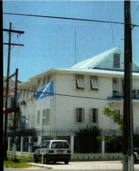
UN Mission, Georgetown, Guyana. Radio facility on roof shows: Verticals x 2 T2FD antenna
