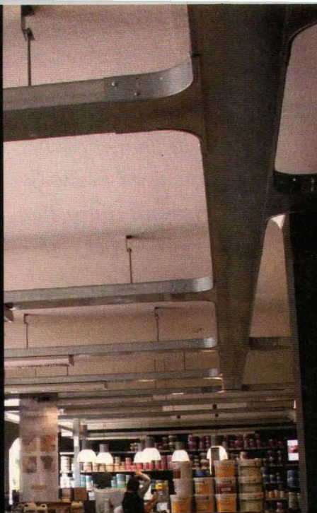
Overhead commercially contained electrical wiring
