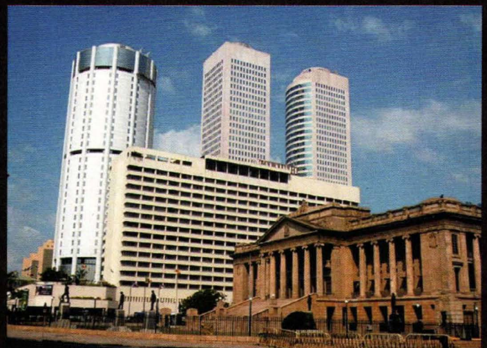
Central Bank Colombo. In 1996 the building was severely damaged by an LTTE truck bomb which resulted in 100 deaths
