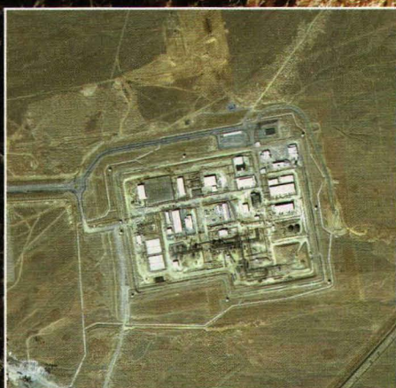
TARGET: The computer programmes which control nuclear facilities such as Arak shown here
