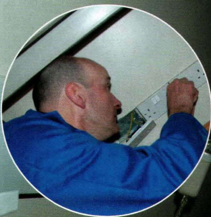
Installing a wired wall socket bug takes a professional just a few minutes
