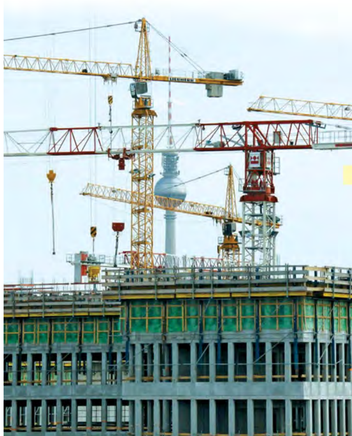
Construction on the new BND headquarters in Berlin began almost a decade ago
