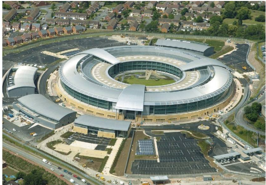
GCHQ new headquarters are readied for its 3500 staffers
