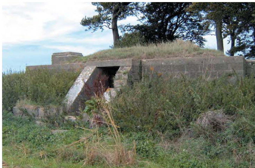
A Starfish decoy control bunker, Liddington Hill near Swindon, Wiltshire. During the Luftwaffe Blitz in WWII, fires were deliberately started at numerous Starfish (SF - Special Fire) sites around the UK to attract marauding bombers away from cities and important facilities
