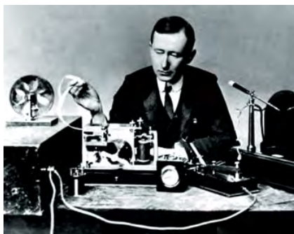
Marconi with his long-distance radio transmission system
