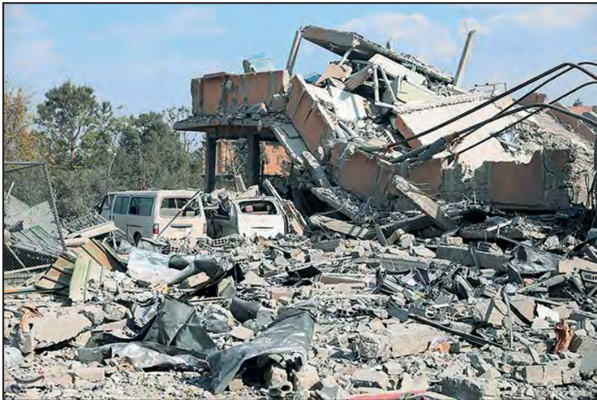
A building destroyed in the allied attack on Syrian WMD sites
