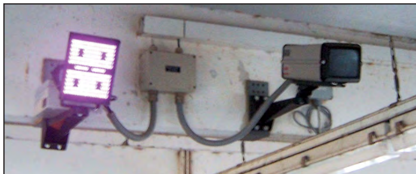
Infrared illuminator. Face recognition technology (including vehicle model and registration plate reader) unit
