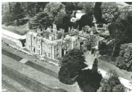
Wartime aerial view of Latimer House near Amersham
