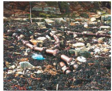
Submarine communication cable probably dating from WWII and defunct, crossing the shore at Hoy, Orkney Islands
