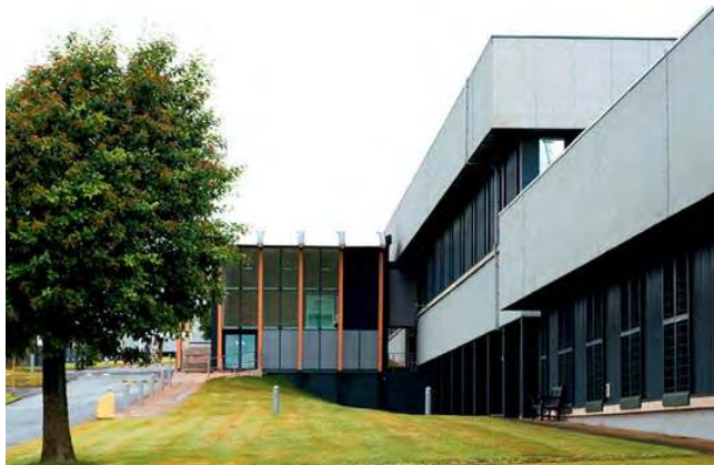
Entrance to GCHQ Scarborough today
