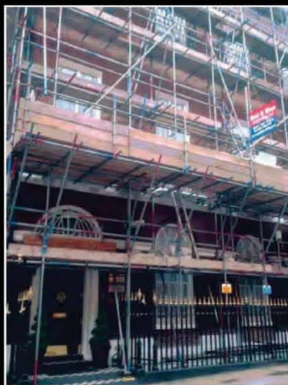
The former GCHQ building on Chesterfield Street
