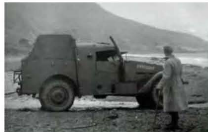
The Poplin Sonic warfare unit mounted on the White scout car undergoing immersion tests, prior to the D-Day landings, believed to be in Ballantrae, Scotland
