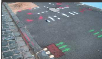
Flags and coloured markers are used to indicate all manner of underground features
