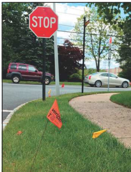
Flags and coloured markers are used to indicate all manner of underground features
