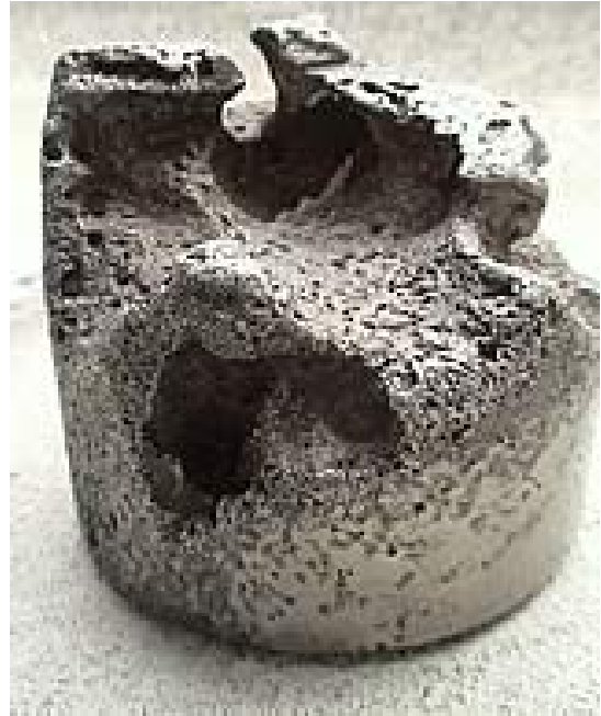
Steel Rod: A close-up of the remainder of a steel-rod, shown disintegrating on TV.
