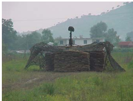
Figure 26: Sandbags Used for Fragment Protection
