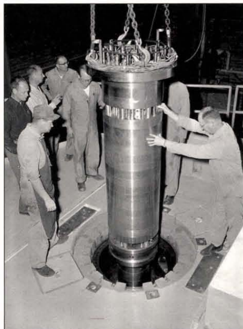
Argonne personnel load radioactive material into the core of EBR-I.
