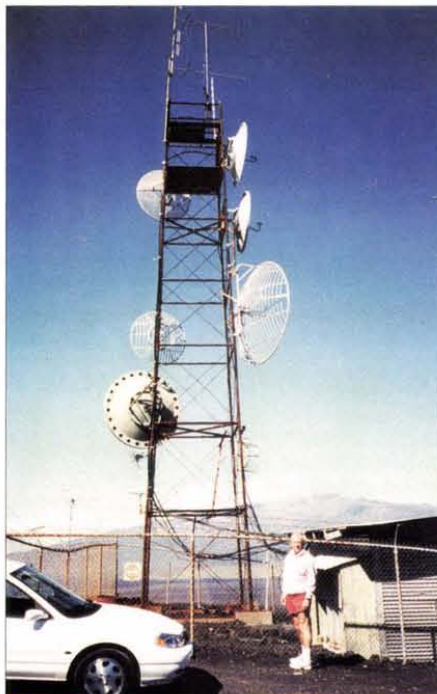
The stacked two-meter Hawaii beacon antennas are at the top of this rusty tower!
